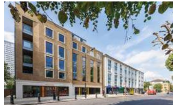
HOLLAND PARK STUDENT ACCOMMODATION
