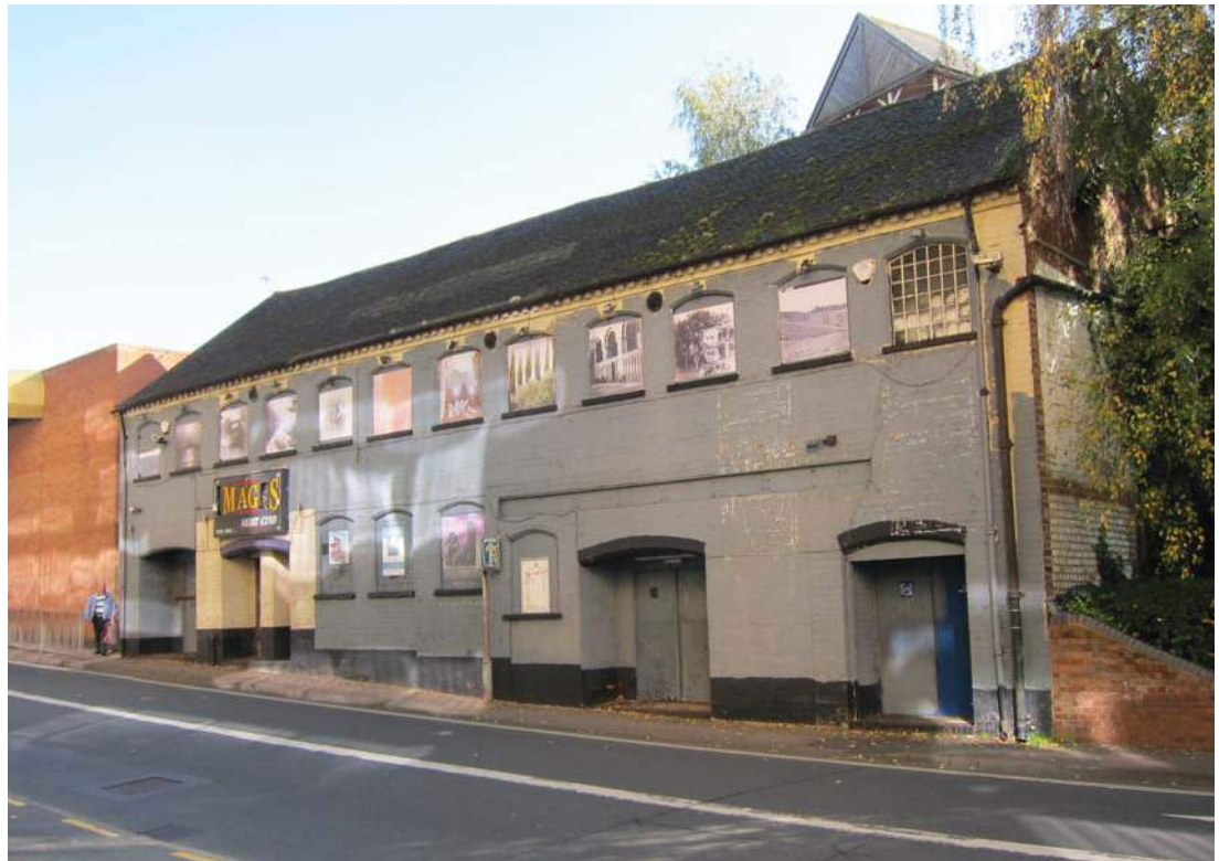
EXISTING BUILDING ON SITE
